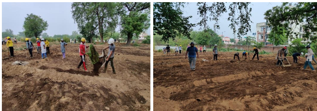
Plantation work at REI site
